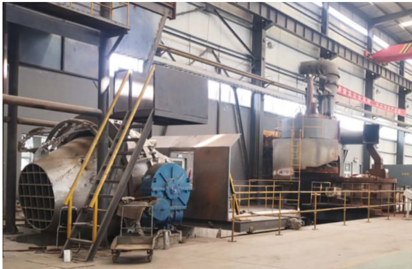
8吨AOD精炼炉 8T AOD Refining Furnace
